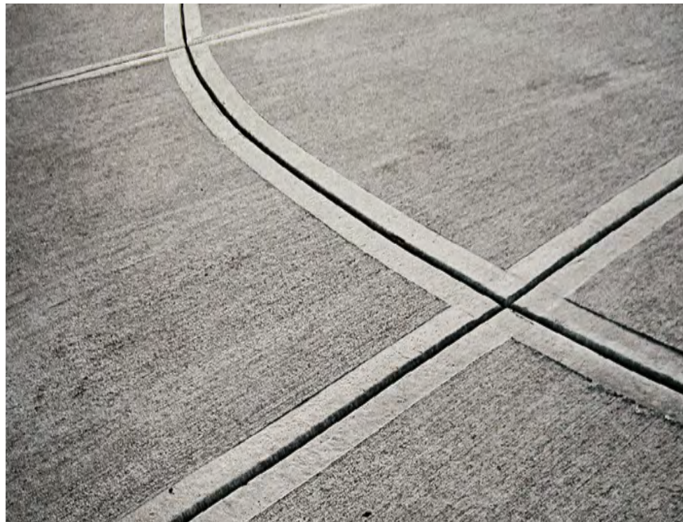
CONCRETE SIDEWALK: 3'x3' Scoring, Hairbroom Finish
