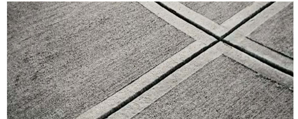
CONCRETE SIDEWALK: 3'x3' Scoring, Hairbrush Finish
